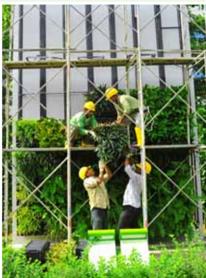
Installation of VGM ®
